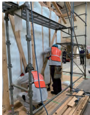
断熱施工の実技講習
