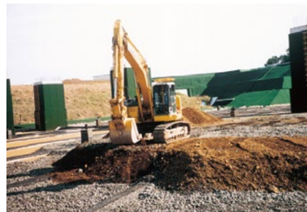
Covering the ash with soil following landfill
