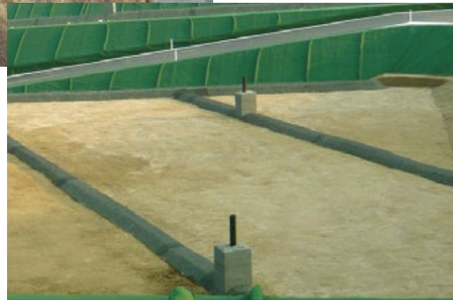
Base section (seepage water collection pipes, exhaust pipes for emitted gases)
