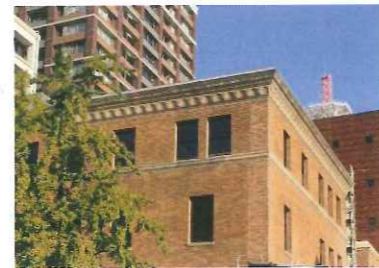
▲外壁や躯体を補修
