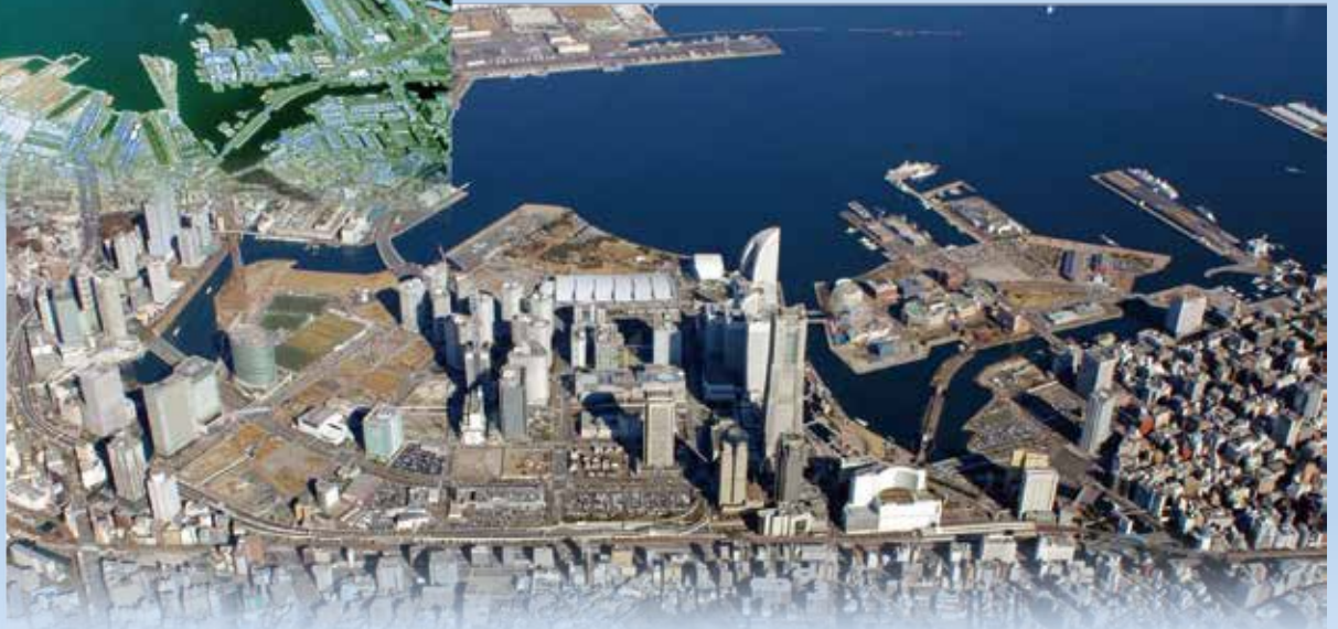
Source: "MINATOMIRAI 21 Information Plans and Projects Vol.84", Urban Development Bureau, City of Yokohama
