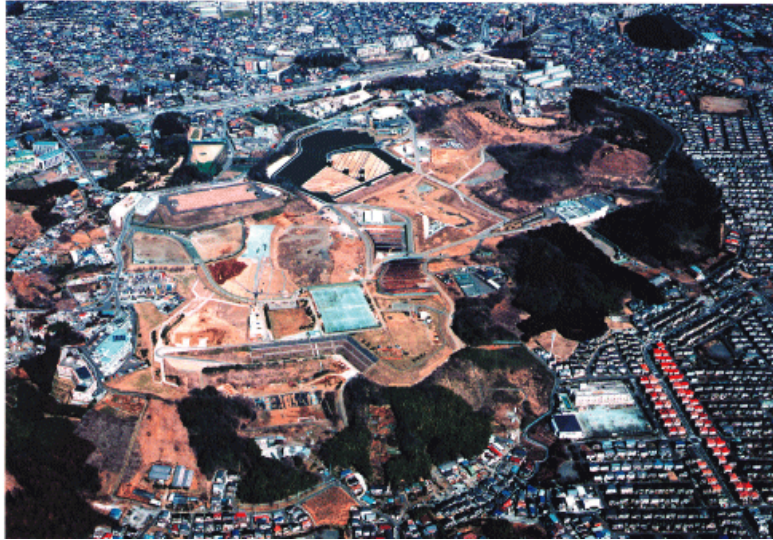
Shinmeidai Disposal Site (1973)
