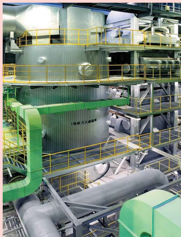
排ガス減温塔・エコノマイザ Exhaust gas cooling tower・economizer
