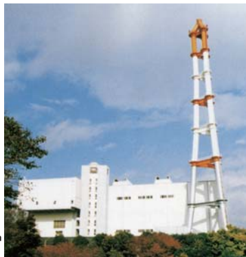
改修前施設外観 Facilities before renovation
