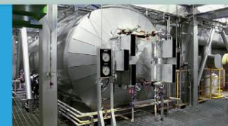
Boilers are facilities that boil water with the heat generated during waste incineration in order to produce steam. The produced steam is sent to steam turbine generators and used for generating electricity. In addition to using this for air-conditioning and water-heating within the incineration plant, it is also distributed to public use facilities that use residual heat to provide a source of heat for heated pools and public baths.
