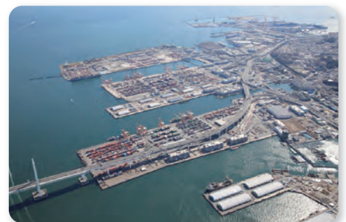
View of Honmoku-Pier
