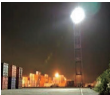
LED lighting in the terminal
