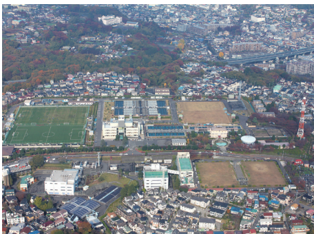
Nishiya Purification Plant
