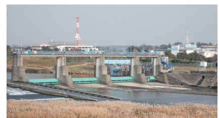
Samukawa intake weir
