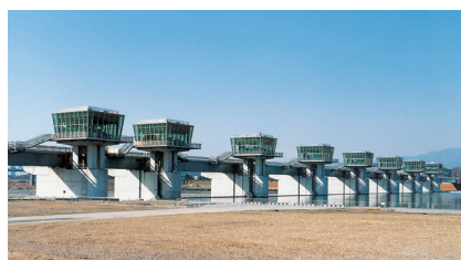
Sagami Ohzeki intake weir
