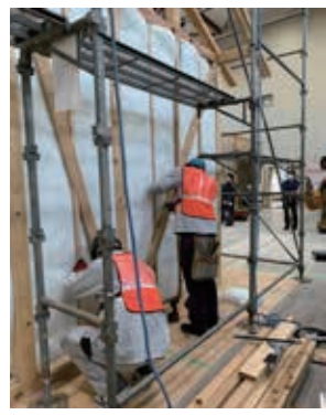
断熱施工の実技講習
