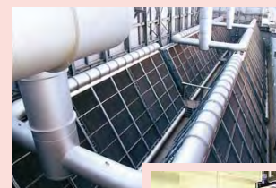
低圧蒸気コンデンサ Low-pressure steam condenser
