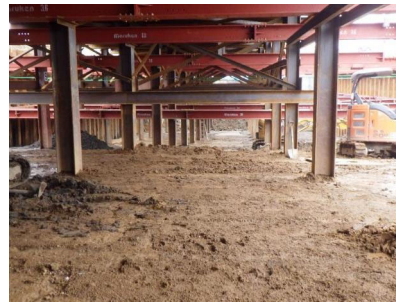
仮設構台下掘削
