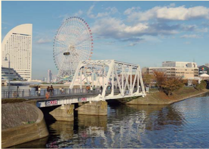
(手前)港一号橋梁 (奥)港二号橋梁
