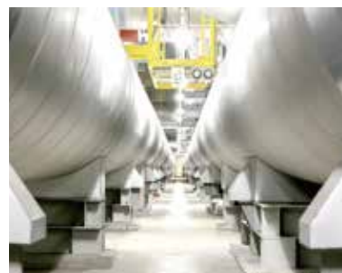
Heat is distributed through pipelines housed in large-scale shared utility tunnels within the district.
