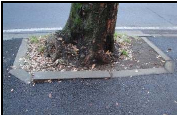
Before work (root lifting & impermeable pavement)
