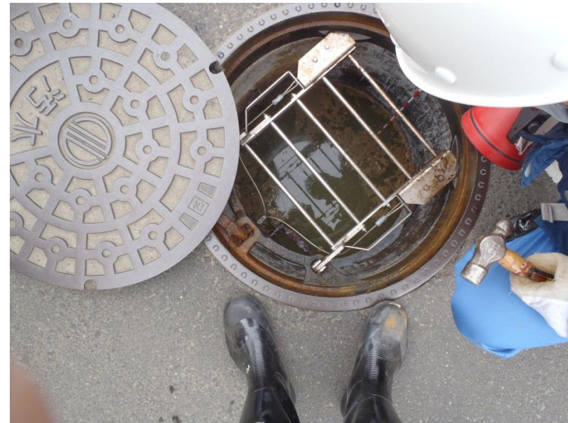
Visual confirmation Inside manholes
