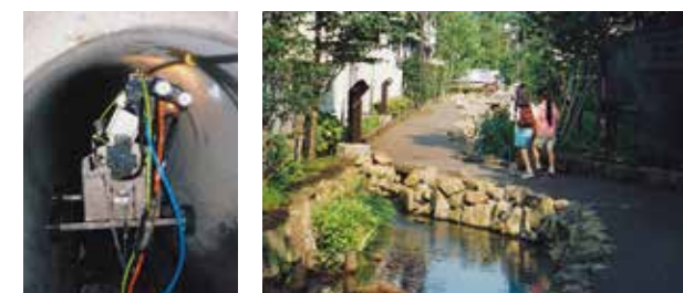
Inside of Sewer Pipe (Optical Fiber Installation) Water from Advanced Treatment (Stream at Irie-River)
