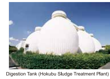
Digestion Tank (Hokubu Sludge Treatment Plant)
