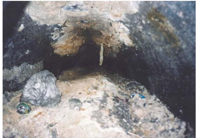
Sewer pipe blocked with oil
