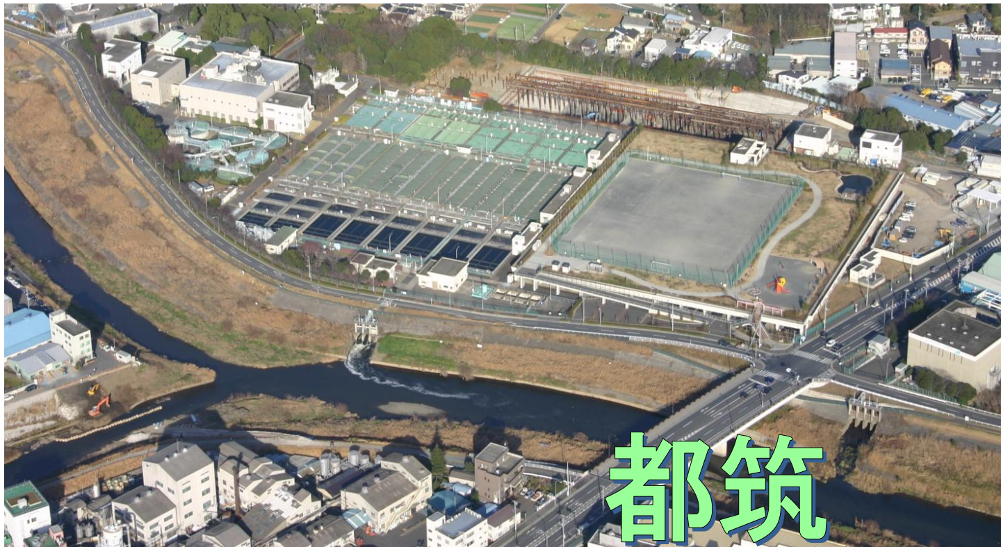
TSUZUKI Wastewater Treatment Plant
