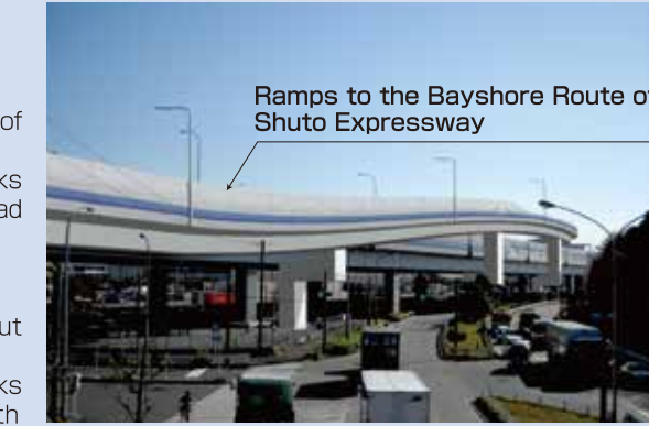
▲Ramps to the Bayshore Route of Shuto Expressway Completion image (The City of Yokohama)
