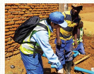
Repairing Leaks in the Republic of Malawi (July 2024)
