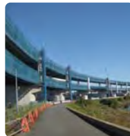
Construction of the Yokohama Loop North Expressway
