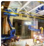
Bridge preservation work
