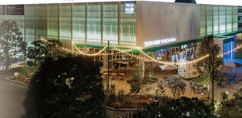
TECH HUB YOKOHAMA (外観)
