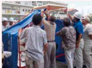
▲ Establishment of a restroom
