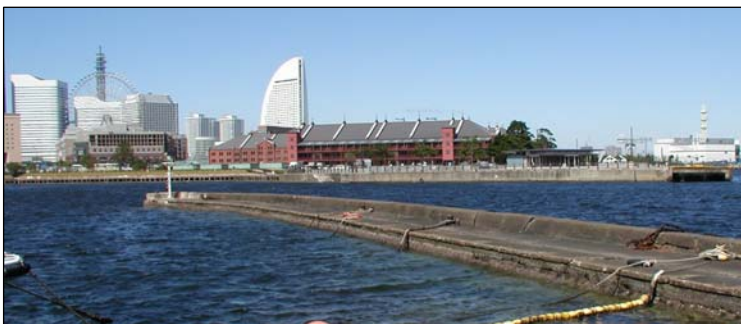
Zonohana, the breakwater, against the Minato Mirai area
