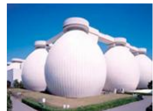
Hokubu Sewerage Treatment Center
